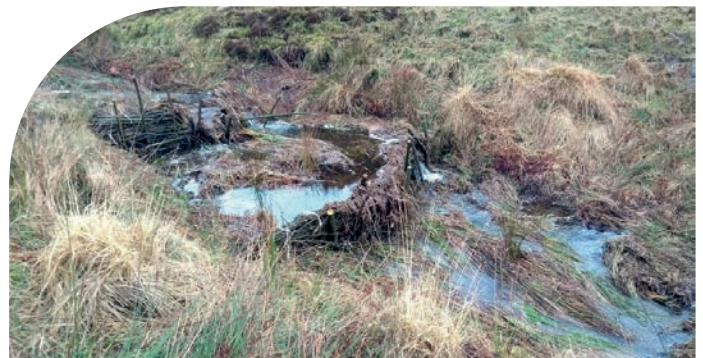
Willow block construction
